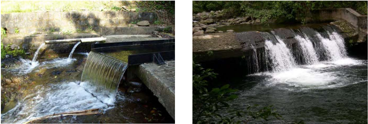
Figure 9. Over hanging diversions on Honopou Stream, Maui (left) and on the middle reach of Waihe'e Stream, Maui (right). Notice how the water free falls and leaves no pathway for upstream migration.
